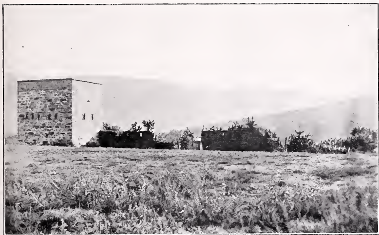
TOWER OF DOUBLE DRIFT FORT
